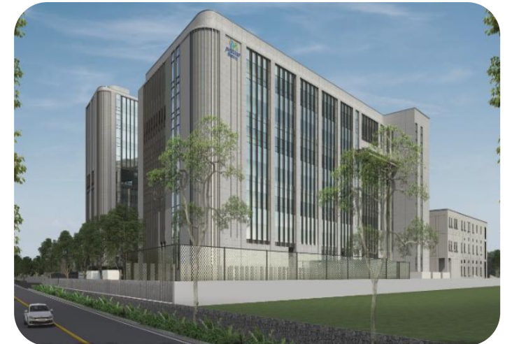
Expansion at new site, Devanahalli, Bengaluru
